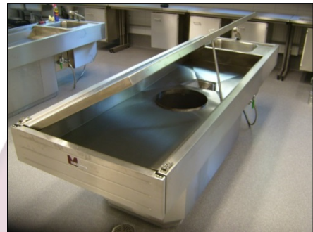
Autopsy table with „Dome“ extraction which we do not recommend. The base of the table is not "one piece" but interrupted with a large hole. This allows water and debris to enter the extraction system, which is a big risk
