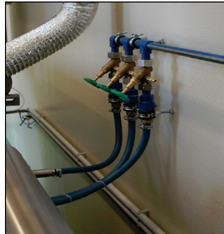
Example for the inlet of a maceration system with 2 chambers (Middle tap for supplying the shower)
