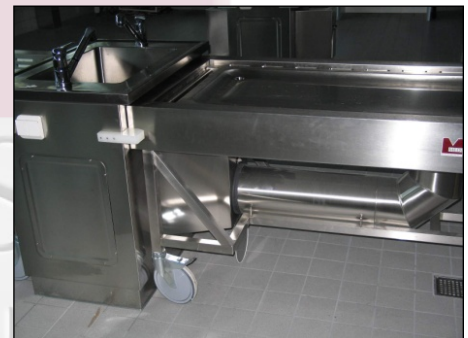
Air extraction duct
