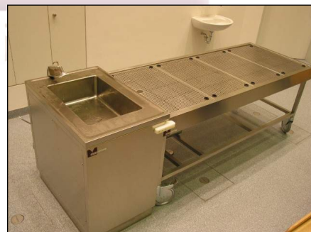
Student demonstration table with extraction connected to a single docking station
