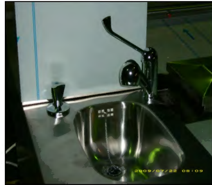
Sink with 25mm radius, elbow operated taps with flexible hose 1500mm long..
