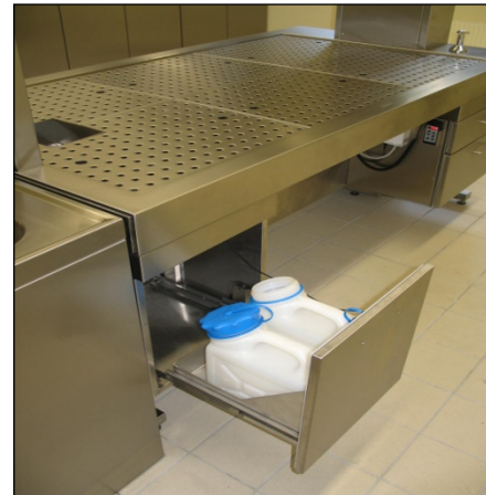
Integrated fresh formalin supply and used formalin drain system
