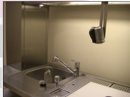
MA-0087 with illumination bridge, camera-holder, sink and duct channel towards ceiling (left)
